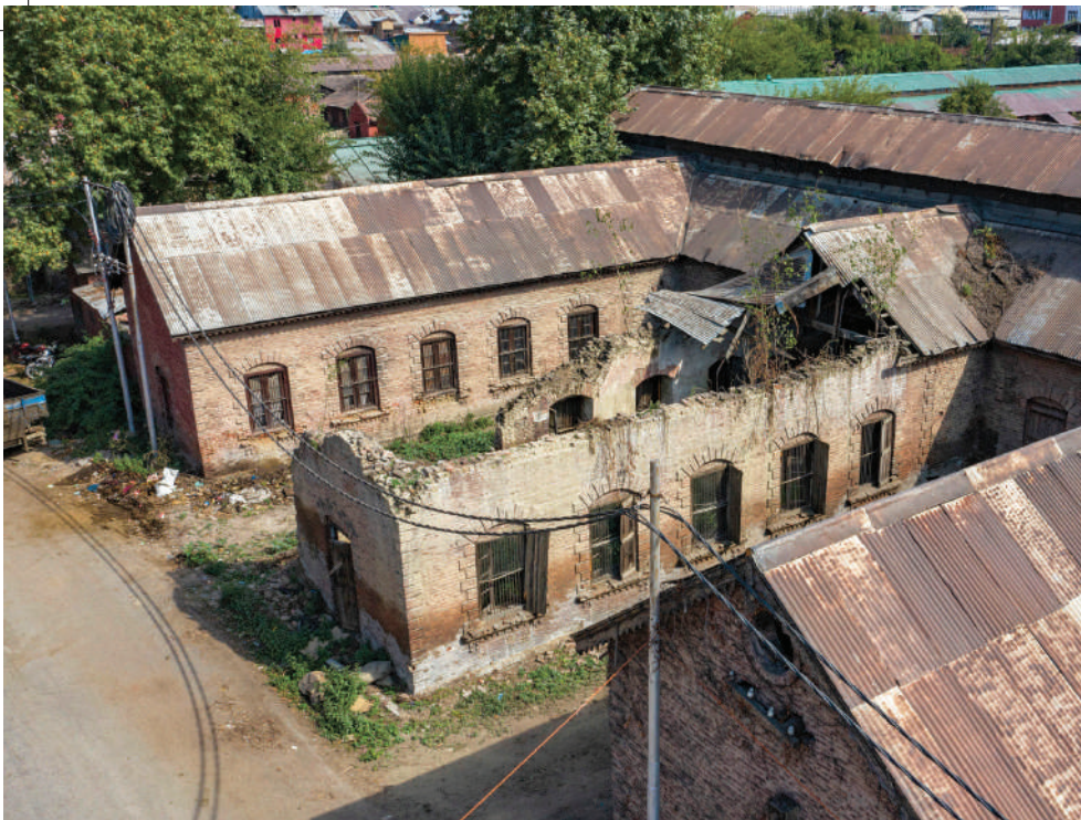
■ Collapsed section of the silk testing building.
