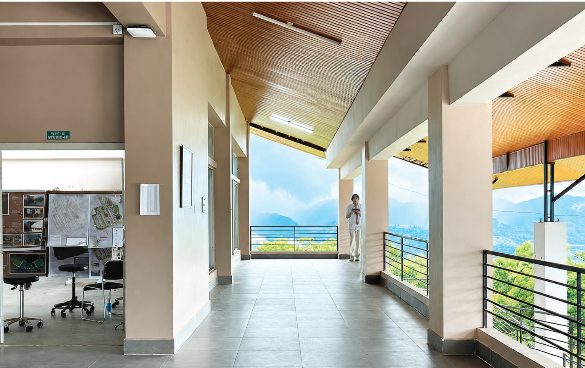
Ample verandah space outside the studios. Corridors and ramps run to the right of the colonnade.
