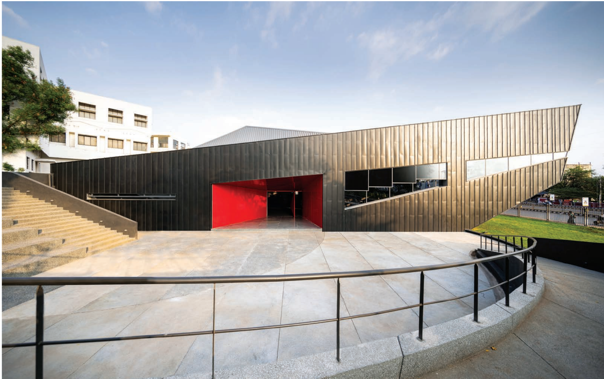
West Plaza and entrance.
