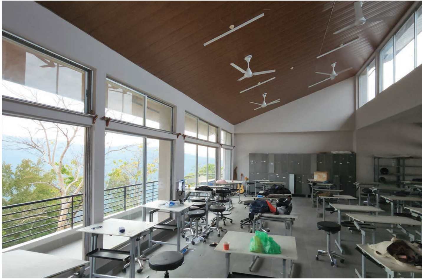
Studio with ample natural light from large windows and clearstory windows. This also facilitates cross ventilation.
